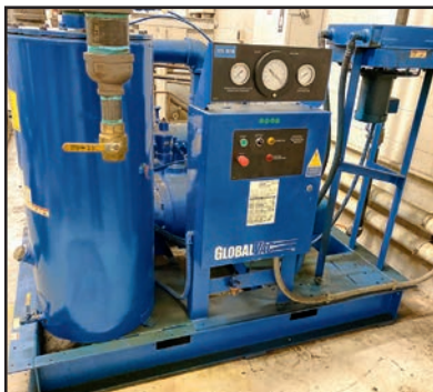
QUINCY QSVI-40 VACUUM PUMP SYSTEM
